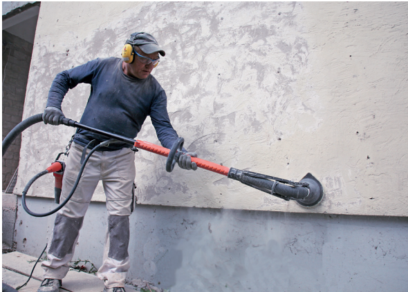
Removing old plaster and paints
