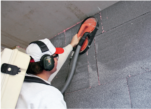
Grinding EIFS and ETICS boards
