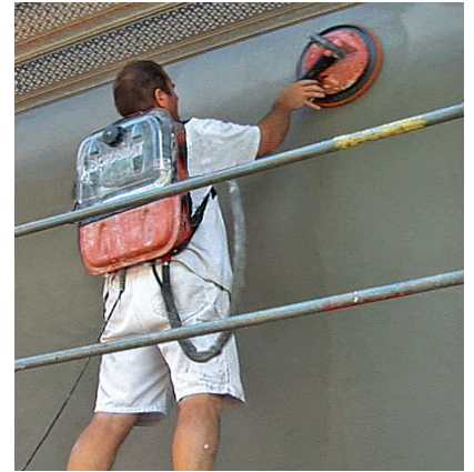
Easy working on scaffolding
