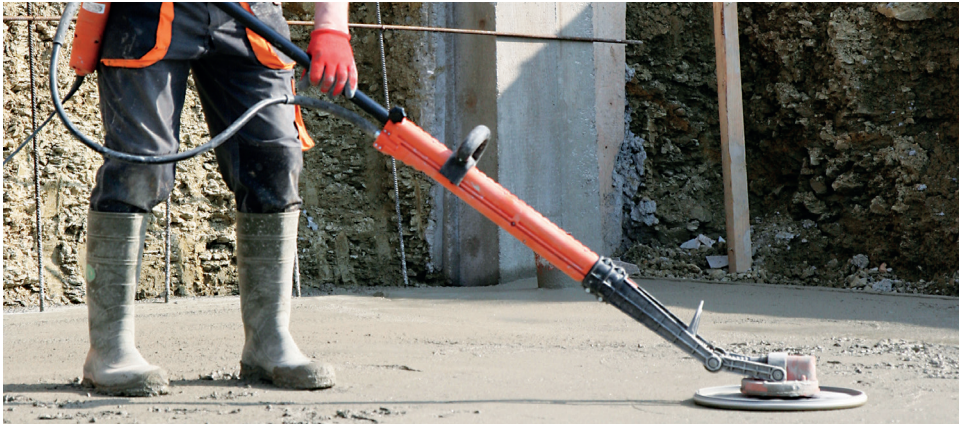
Levelling fresh concrete
