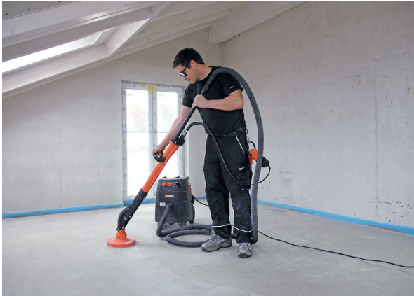
Grinding screeds
