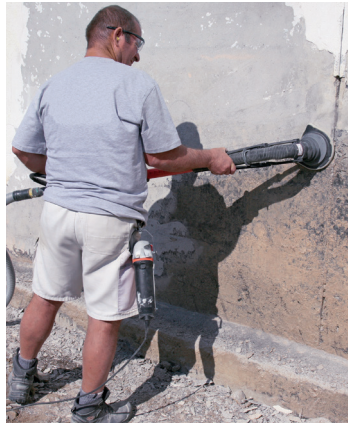
Grinding bitumen coating with PCD grinding disc
