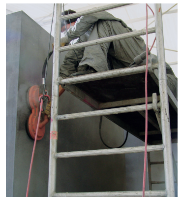
Polishing fair-faced concrete
