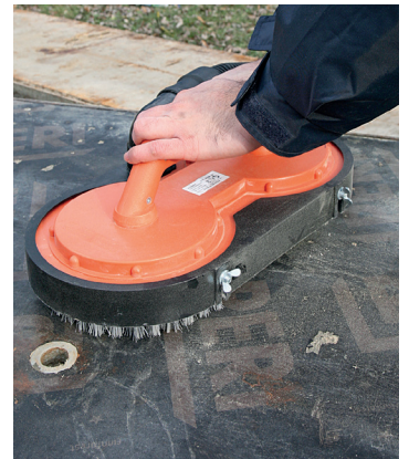
Cleaning formwork units
