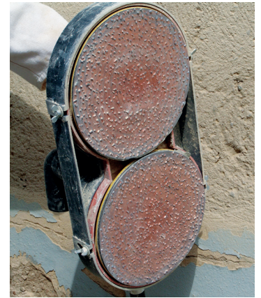
Removing old plasters
