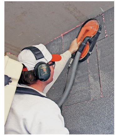
Grinding EIFS and ETICS boards
