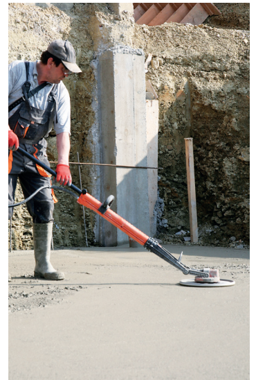
Levelling fresh concrete
